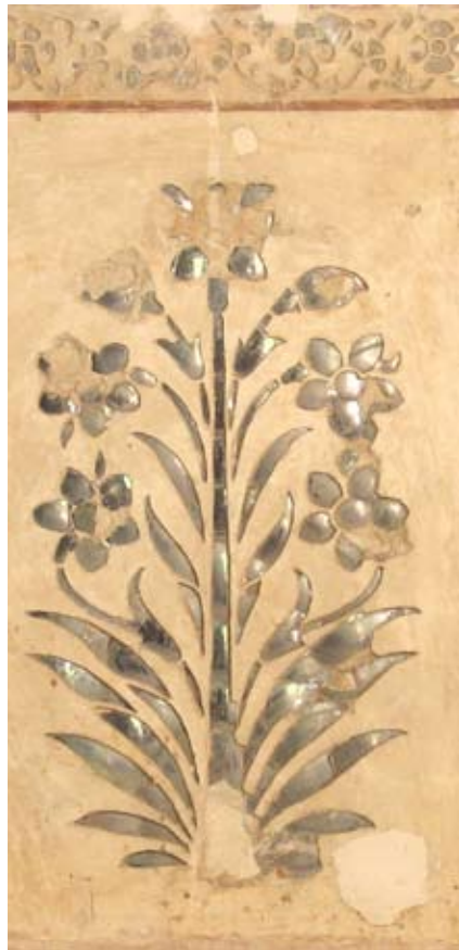
Left: the lower dado in the Sheesh Mahal is decorated with grey-blue inlaid mirror-work. The mirror is a sodium-based silica glass, (see EDS spectra of Sample #3806 above) with a lead foil backing. In the back-scattered SE micrograph (40x) of Sample #3806 below, the lead foil is imaged as the white layer.
