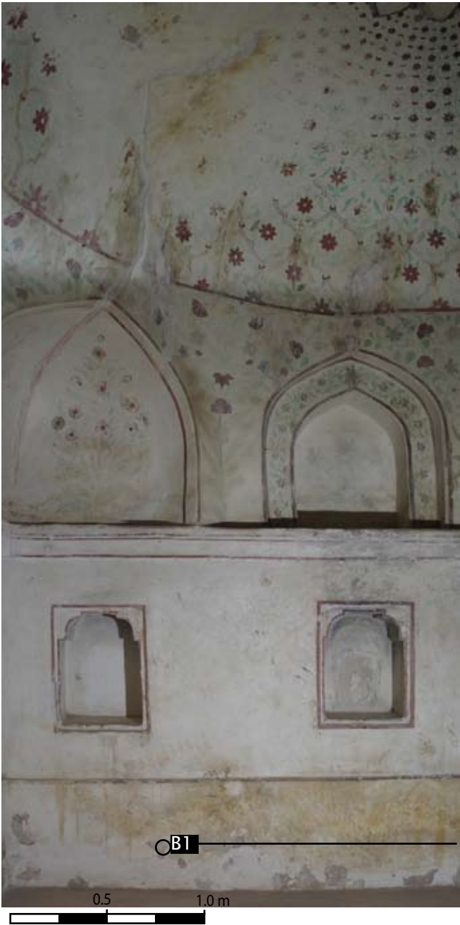
Loss in original plaster; some salt efflorescence (H: 0.24 m)
