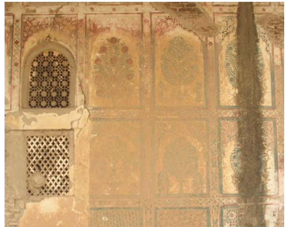
Left: view of the East façade of the Abha Mahal. Above: the painting scheme on the East façade is obscured by a heavy deposition of dirt.
