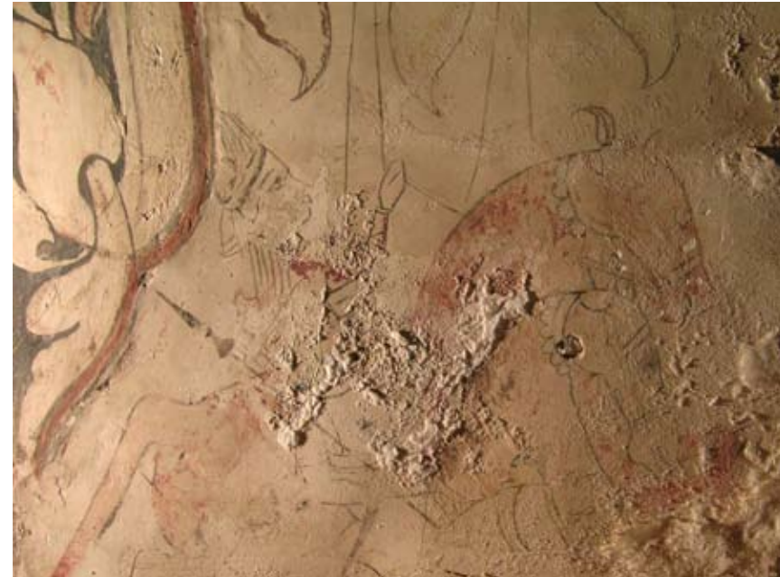
Above: area of salt efflorescence from Room 10, the Abha Mahal. Below: SE micrograph (secondary electron, 700x) of salt sample (Sample # NAG05-26-11) from the area illustrated above in the Abha Mahal.
