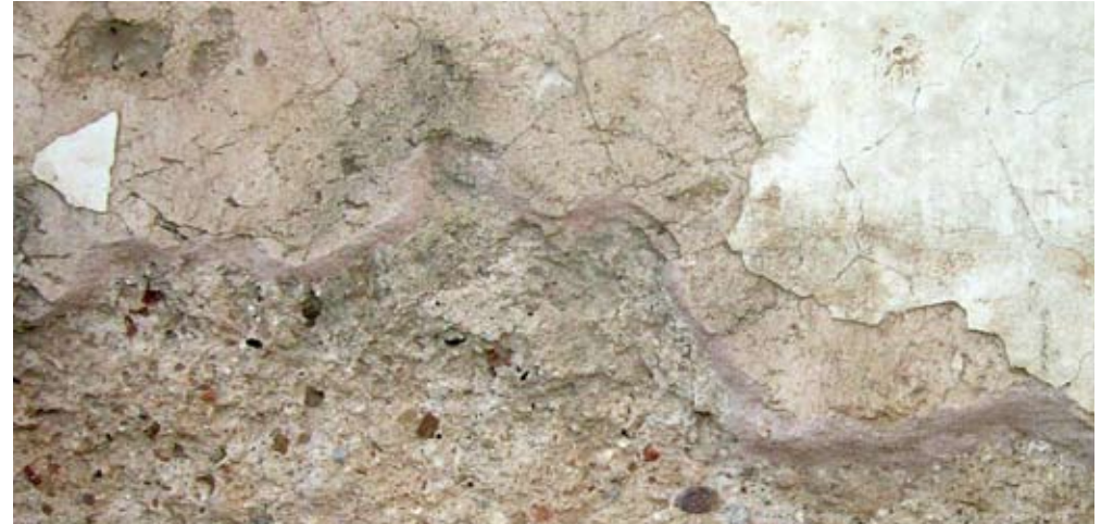
Above: an area of exposed detached plaster on the north facade of the Hadi Rani Mahal before (above) and after (below) the application of a trial edge repair.
