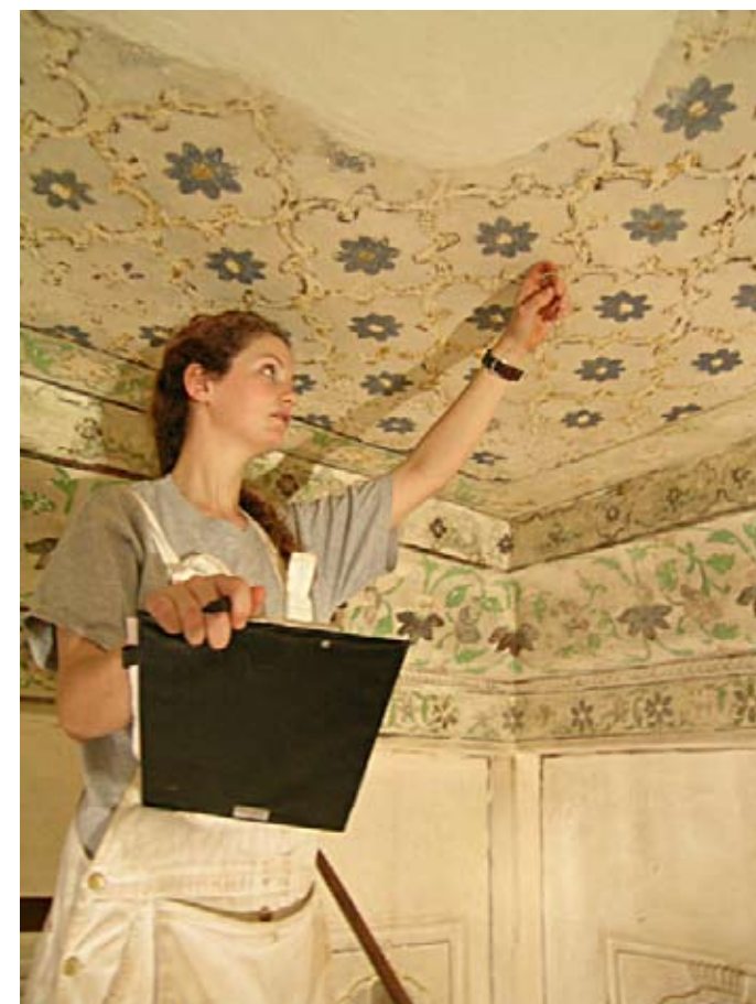
Above: documentation of the detached plaster in the Bakht Singh Mahal being undertaken by Sibylla Tringham (Courtauld Institute).
