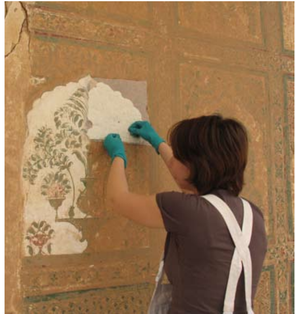
Above: Stephanie Bogin (Courtauld Institute) applying a sorbent during cleaning trials to remove the heavy deposition of dirt which obscures the exterior scheme on the east facade of the Abha Mahal.
