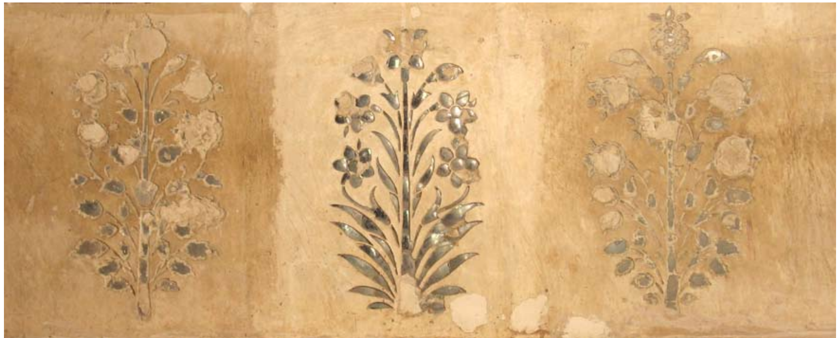
Left: a cleaning trial in Hadi Rani Mahal, first floor, after removal of a discoloured synthetic coating.
