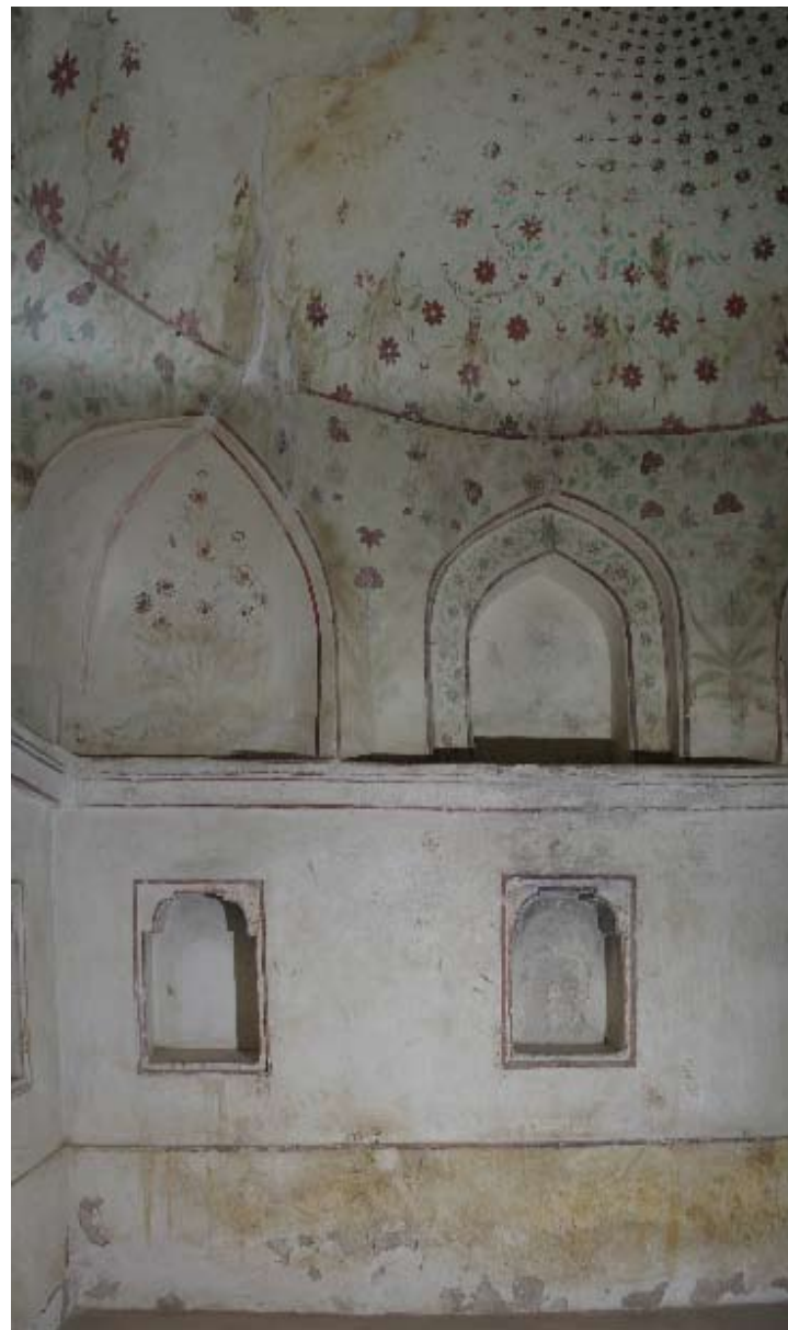
South wall of the Hammam showing brown staining and pigment loss in the dome area, and plaster loss at ground level. Sample B1 was taken from this wall.
