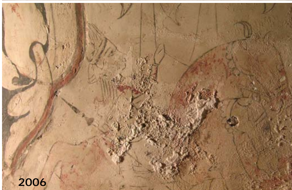
Above: an image of an area with salt-related deterioration in Abha Mahal room 10 taken in September 2005, Below: an image of the same area in March 2006, showing loss due to ongoing salts activity.
