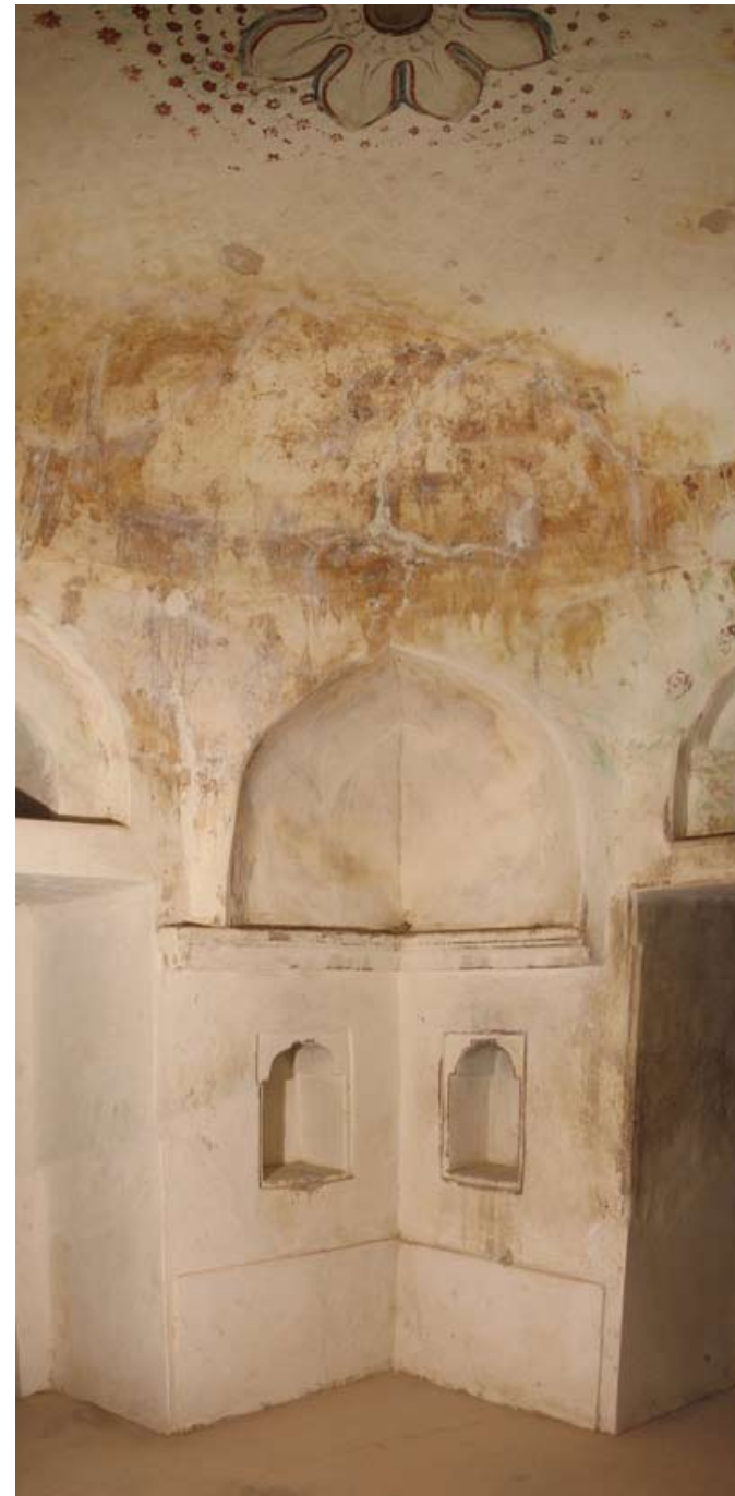
The north-east corner of the Hammam shows evidence of water infiltration: staining, plaster loss and salt efflorescence. This area was chosen as a sampling location for the liquid moisture investigations to determine if infiltration continues in the Hammam.
