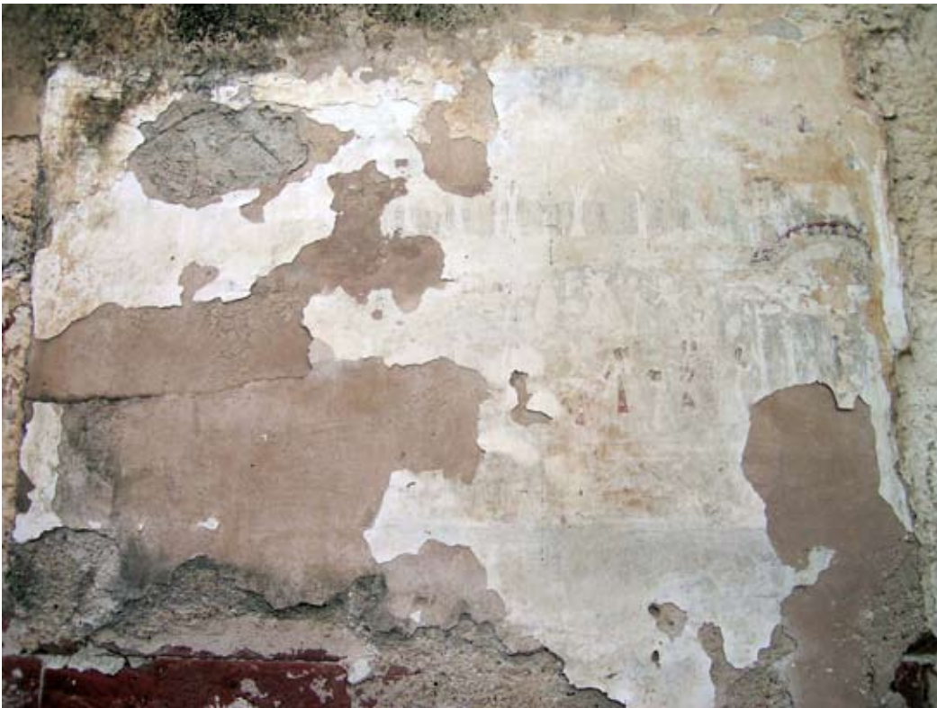
Above: the fragmentary remains of a severely detached painting on the north façade of the Hadi Rani Mahal before facings were applied.
