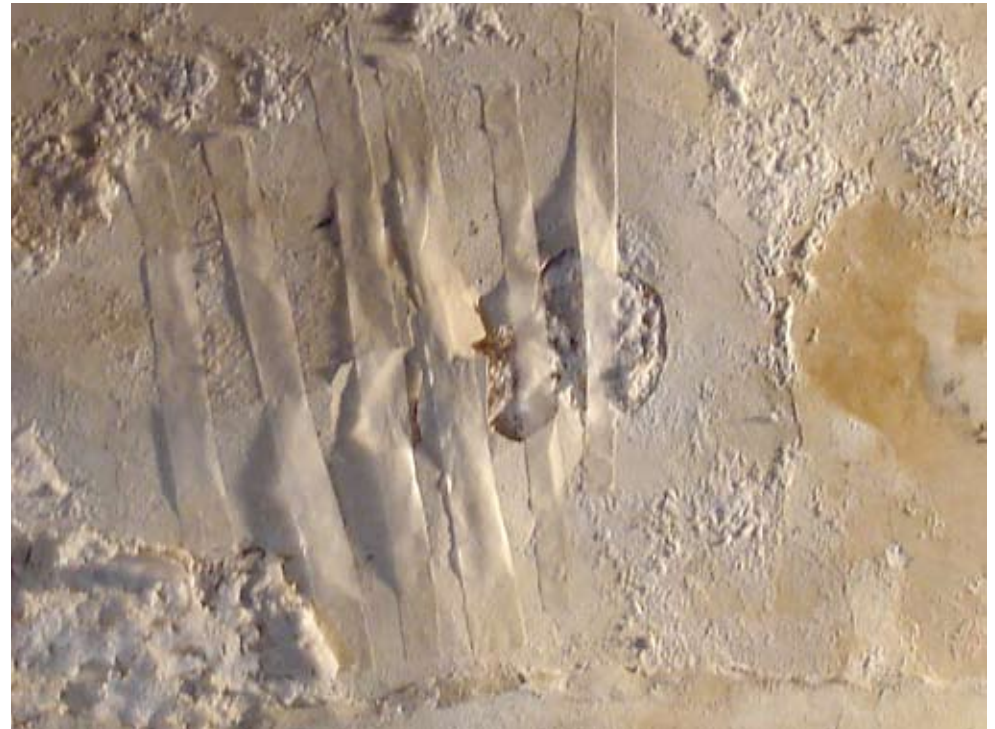
An area of severe detachment due to salts activity in room 10 of the Abha Mahal: before (above) and after temporary facings were applied (below).
